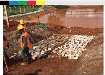
MCPY 15 - Stone pitching work-outlet of the sedimentation pond
