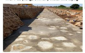
MCPY 15 – ongoing stone masonry for approach slab
