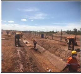
MCPY9 Area 1b: Soil Crete lining at perimeter ditch
