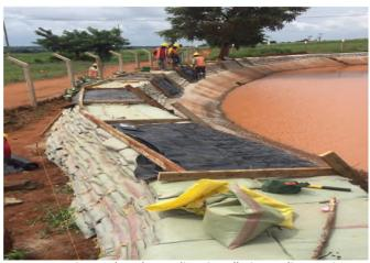
MCPY 15 - Wire mesh and HDPE liner installation-Sedimentation
